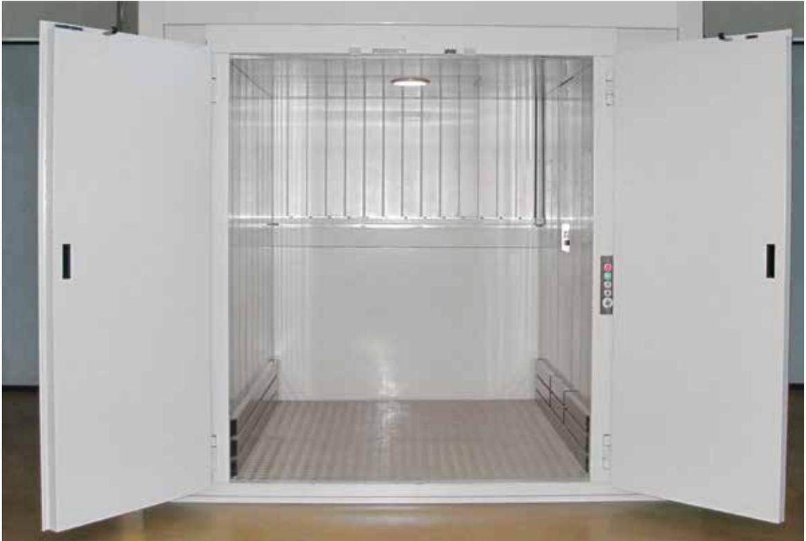
The **Pitless** solution, for VRC and material lifts type B. This system is specially designed for buildings whose facilities have architectural restrictions need, to adapt to local regulations, to save potential problems of water infiltration and for situations where a pit is not feasible.
