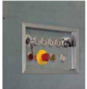
Recessed COP (Car Operating Panel) with hold-to-run push button, protected by a frame to prevent damage during loading operations.
