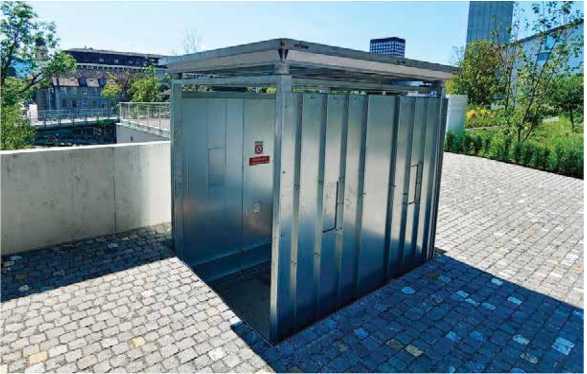
Lifts with inverted slings are used when guides must not protrude from the floor at the last stop. The upper floor itself must be flat and free of any obstacles while the lift is not in operation (stages, heliports, etc). For each of these applications, specific safety measures must be taken and a qualified person must operate the good lift.
